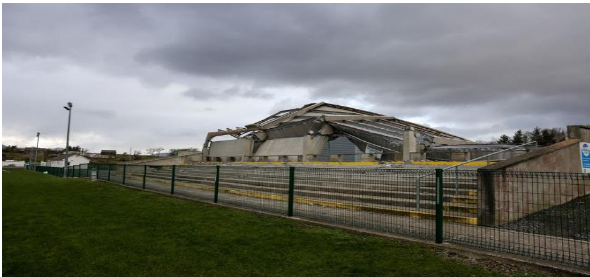
Severely damaged stand at Burrishoole GAA Club
